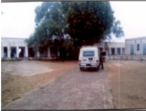
Building Front View
