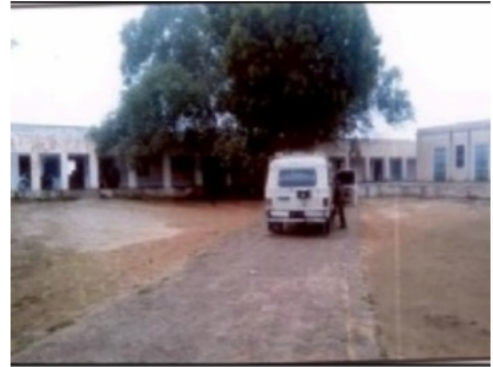
Building Front View
