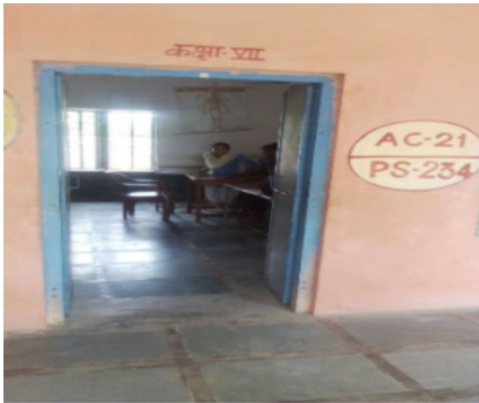
Polling Station Building Front View
