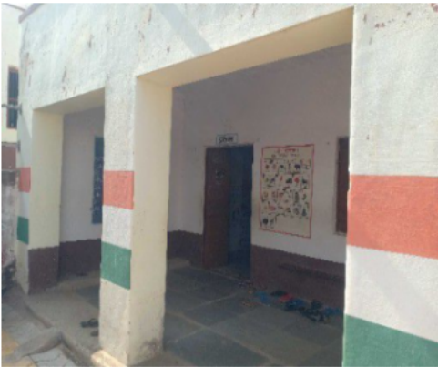
Polling Station Building Front View
