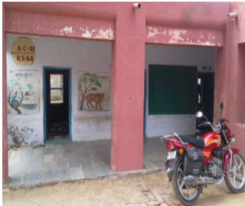
Polling Station Building Front View
