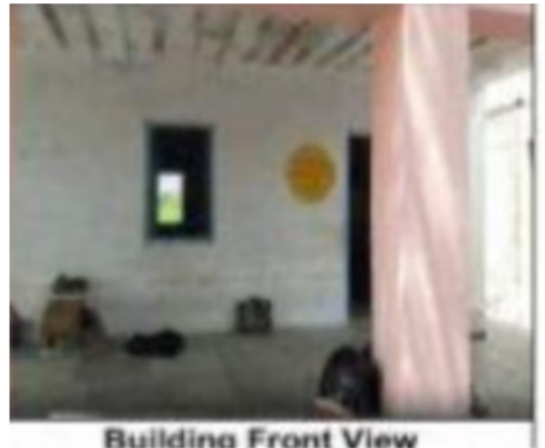
Building Front View
