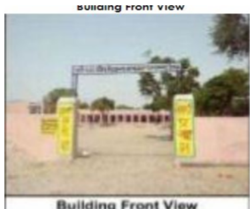
Building Front View
