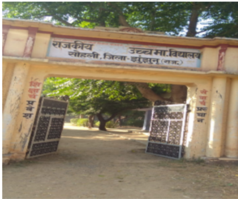
Polling Station Building Front View
