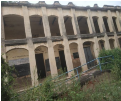
Polling Station Building Front View
