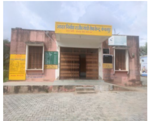
Polling Station Front View
