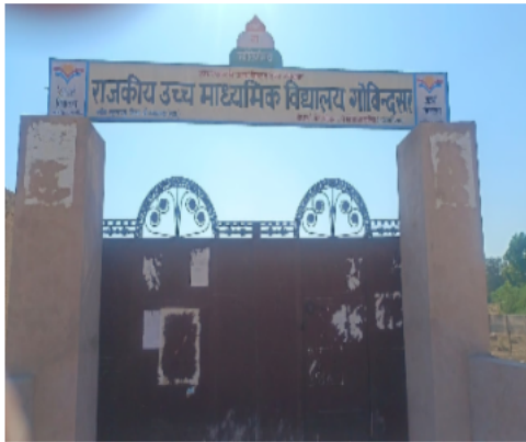
Polling Station Building Front View
