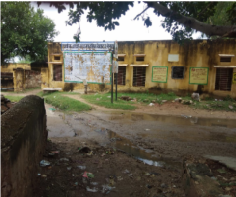
Polling Station Building Front View
