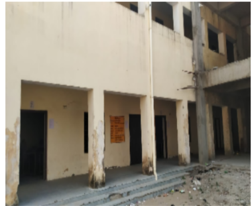
Polling Station Front View
