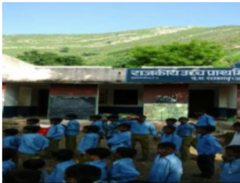
Building Front View
