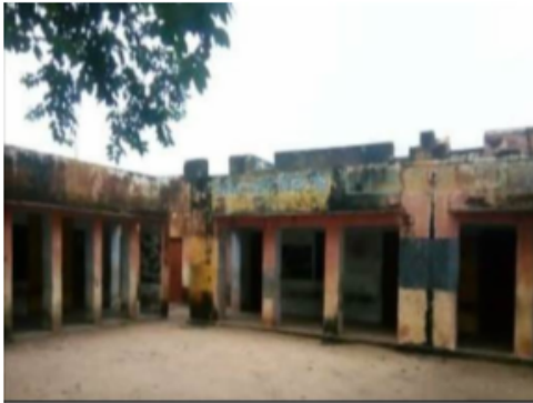
Building Front View
