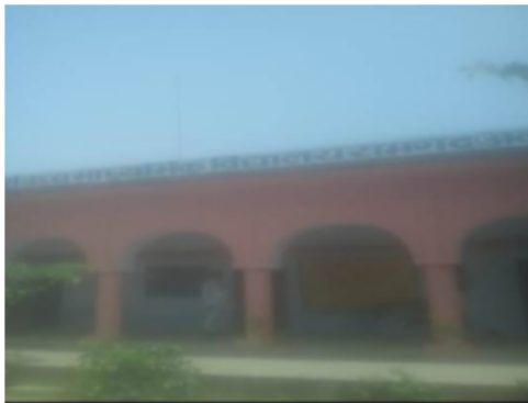
Building Front View
