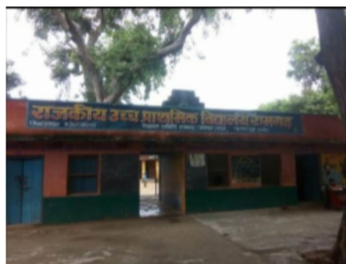
Building Front View
