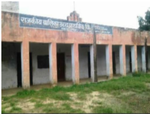
Building Front View
