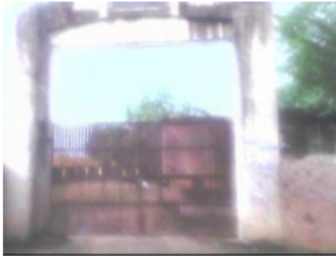
Building Front View
