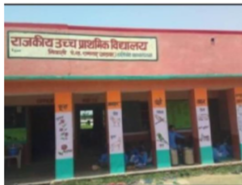
Building Front View
