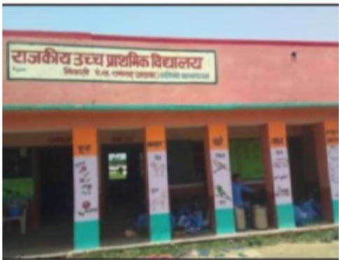
Building Front View
