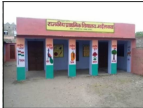
Building Front View
