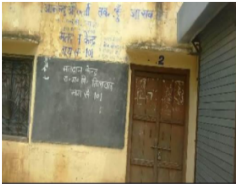
Building Front View
