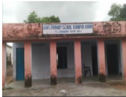
Building Front View
