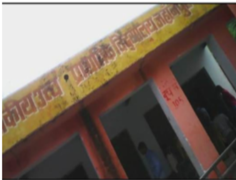
Building Front View
