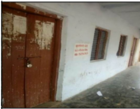
Building Front View
