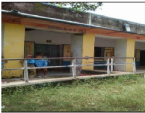
Building Front View
