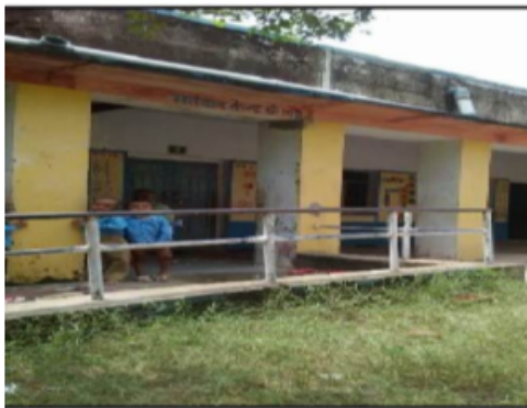
Building Front View
