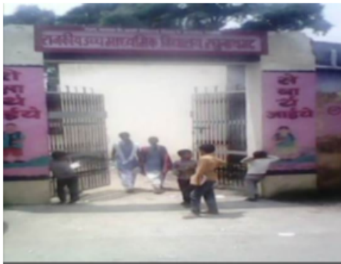
Building Front View
