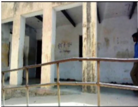
Building Front View
