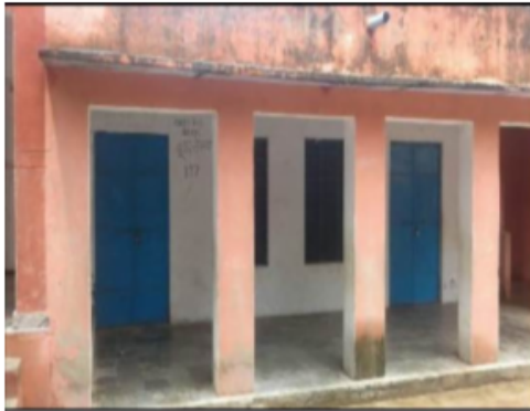
Building Front View
