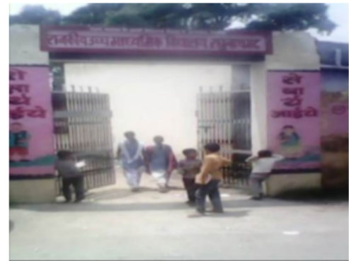
Building Front View
