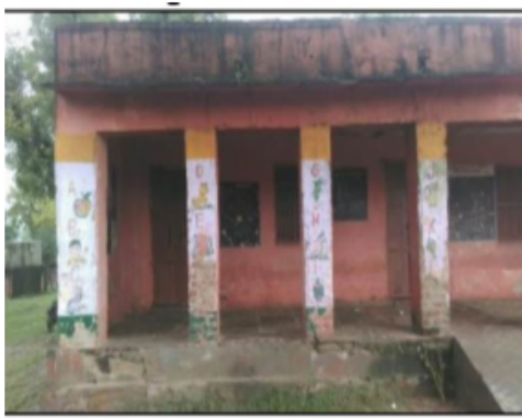
Building Front View
