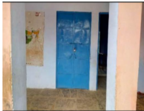
Building Front View
