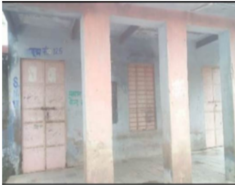
Building Front View
