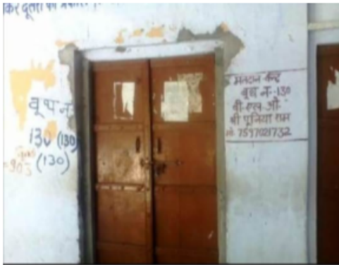
Building Front View
