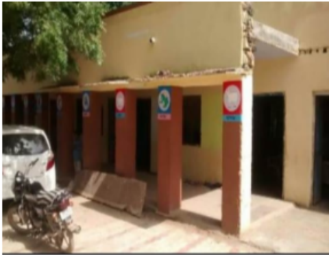
Building Front View
