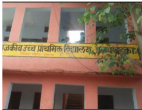
Building Front View
