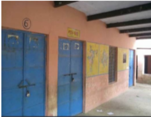
Building Front View
