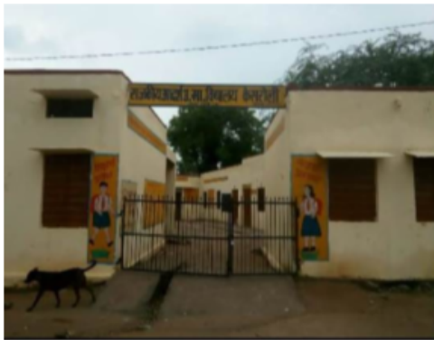
Building Front View
