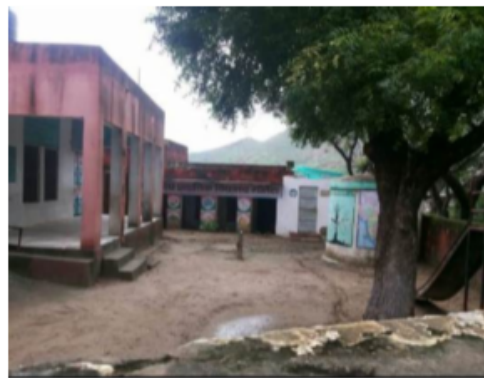
Building Front View
