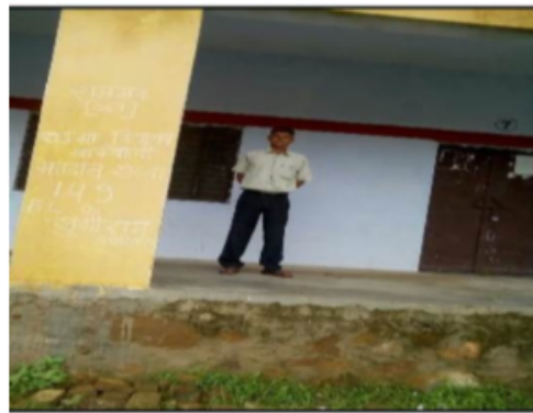
Building Front View
