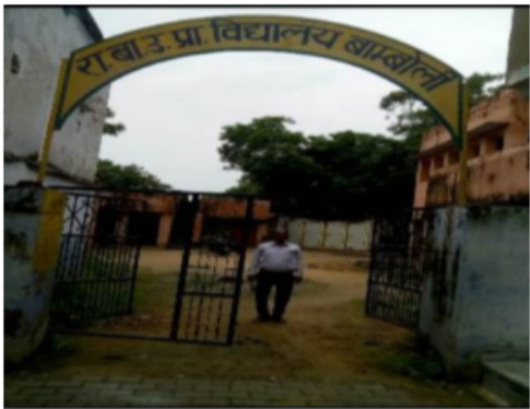
Building Front View
