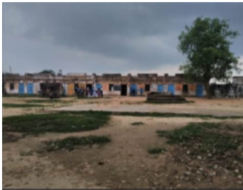
Building Front View
