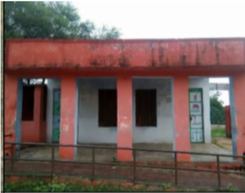
Building Front View
