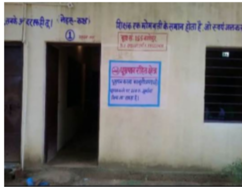
Building Front View
