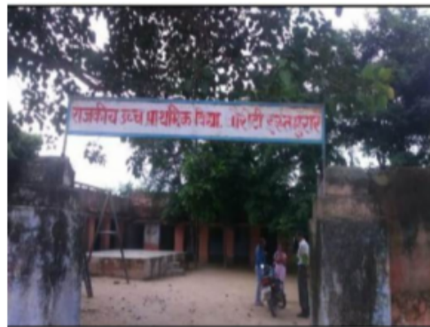
Building Front View
