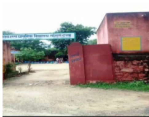
Building Front View
