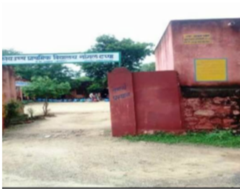
Building Front View
