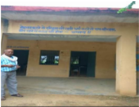
Building Front View
