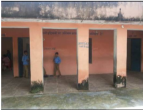
Building Front View
